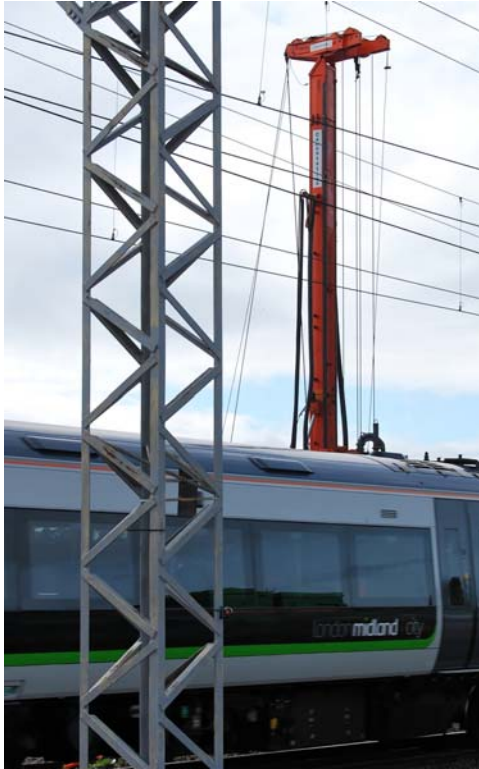
Pictured above: A piling rig works close to the busy West Coast mainline whilst the Leica equipment and GeoMoS software monitor the track for movement.
